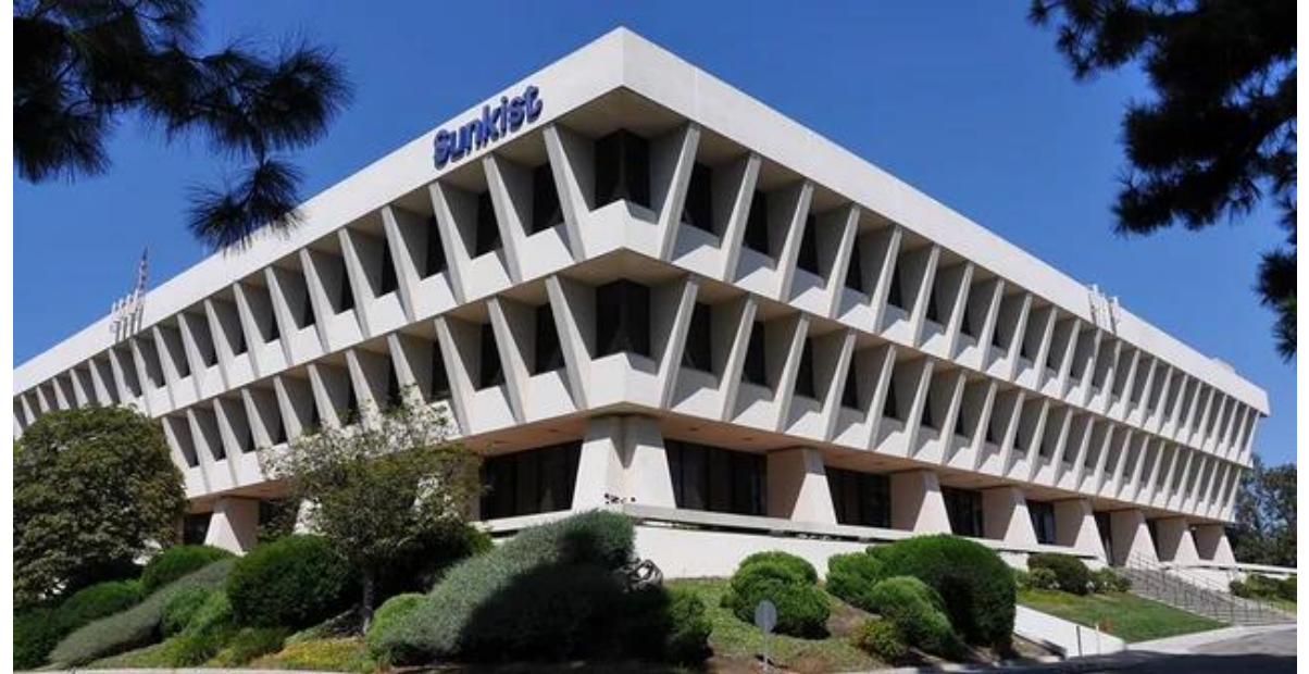
Sunkist Headquarters 14130 Riverside Drive
