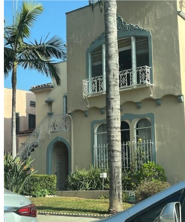
Existing homes across the street
