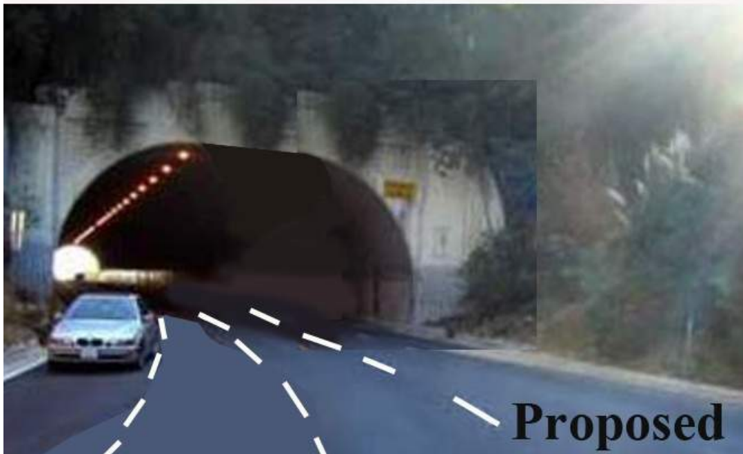
Enlarged Mulholland Tunnel
